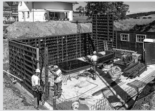
Wall formwork
