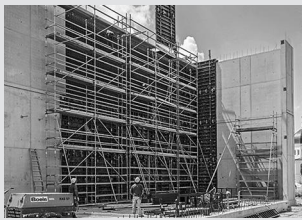
Working scaffolds construction
